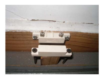
• In this installation example, the Contact Element is mounted above the garage door (on the door frame), at a height that ensures unobstructed door motion (the garage door's tracks begin pulling the door away from the frame by the time the top edge of the door becomes parallel to the Contact Element). The Magnetic Element is mounted on the top edge of the door, at a height that places it within the required distance and alignment of the Contact Element when the door is fully closed:
