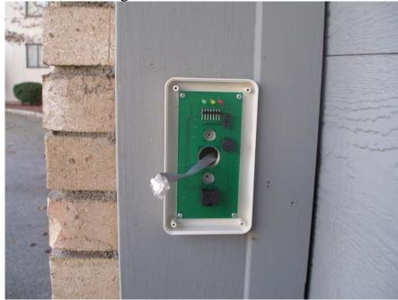
• 5. Connect the network cable to the Circuit board and pull the excess cable back through the door frame.
